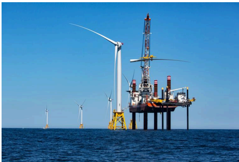
Figure 1: The Block Island Wind Farm under construction [5]
